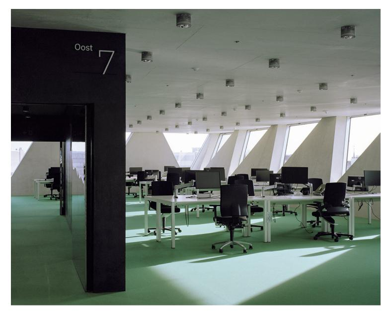
The building is conceived as a bridge structure over and across the pavilion. At the center of the plan, one large steel truss spans from one core to the other. Two more trusses are integrated in the concrete side walls and their triangulation defines the form of the window openings. In a next step, this window form is applied all over the building as it provides maximum efficiency in striking an ideal balance between daylight access and overheating by the sun. The opaque façade is clad in
