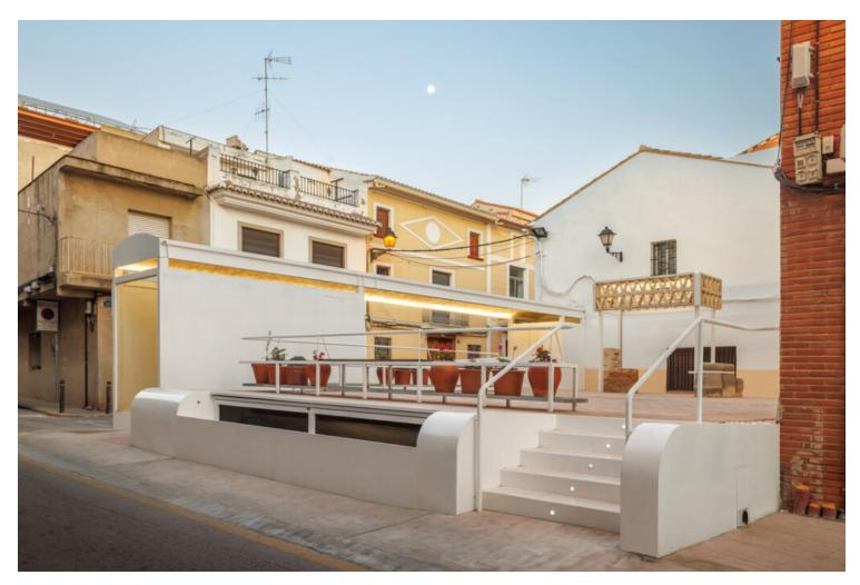
Built using a combination of industrialized construction and traditional techniques, a ceramic lattice sits atop a structure of metal profiles that recovers the idea of the original "turret". Some of the pieces found during the excavations, subsequently restored, such as the manual wheel pump and pieces of the fountain's basin, are installed beneath it.
