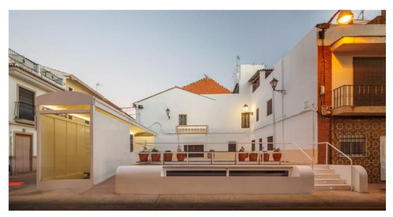
The square, bounded by the adjoining façades, occupies the area above the cistern, rising some 90 cm above street level in order to recover the full span of the vaults in the space below. An observation point is installed at the front of the square that provides views of the remains of the cistern from street level.
