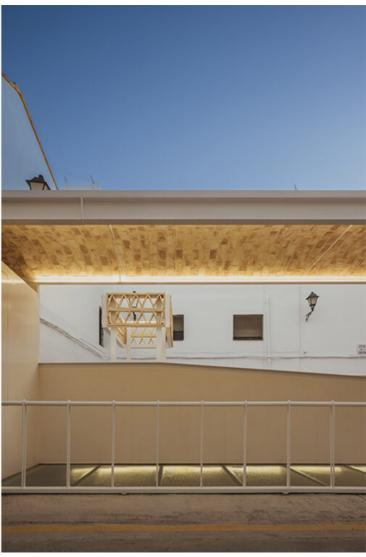
Above ground, the design uses two materials: steel and ceramics (tile and brick). The intention behind the use of these materials is to provide for a reversible, dry construction while also incorporating a local material that blends into the urban environment of the Vila, rooted in the Valencian building tradition, and which generates a sense of familiarity among users.
