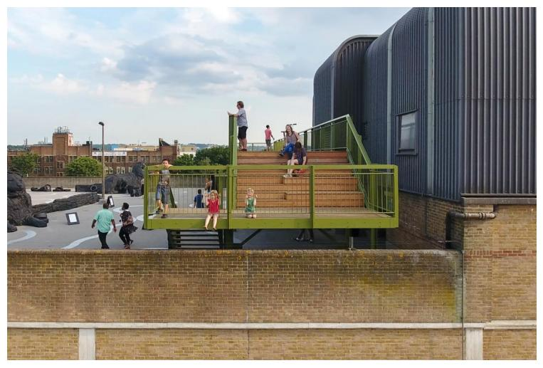
For Bold Tendencies, their 3.5m-wide raised platform spans the entire width of the car park, its steel support beams cantilevered at both ends. Two staircases at either side provide an elevated promenade, and on the northern tip the balustrade position at the half-landing provides unencumbered views of London.
