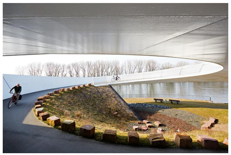
The combination of design strategy and safety requirements has resulted in a bridge with an elegant, curved and sculptural form. The construction, with a total length of approximately 170 m, consists of a continuous five-part girder, which allows some 70 m to be spanned at the harbor entrance. Viewed from above, the bridge appears as a lightly undulating S-shape, which, at its north end, culminates in a circular access ramp: a 14-meter spiral, constructed of white concrete. On the
