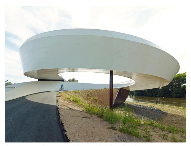
The oil depot is used for the transfer and storage of highly flammable substances. For this reason, the bridge had to be designed to prevent people on the bridge from gaining access to the passing tankers, or at least to make it difficult. In view of these exacting circumstances, a solution was developed that not only fulfils all the safety requirements, but also takes into account the specific location of the bridge on the Main River.
