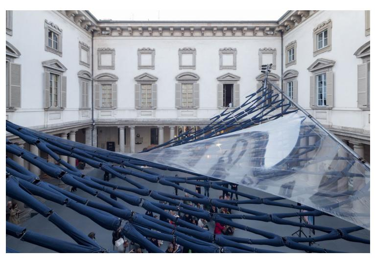
The roof canopy is composed of 300 pairs of jeans. Deploying the jeans as a ready-made, intentionally mis-using and translating them from the context of the human body into an architectural module. The design exploits the implicit structural logic of the jeans—connecting them waist-to-waist and cuff-to-cuff—to create a tensile, catenary diagrid that spans the open space of the courtyard. The net gives the impression of a body imprinted in space, but one also de-familiarized by repetition.
