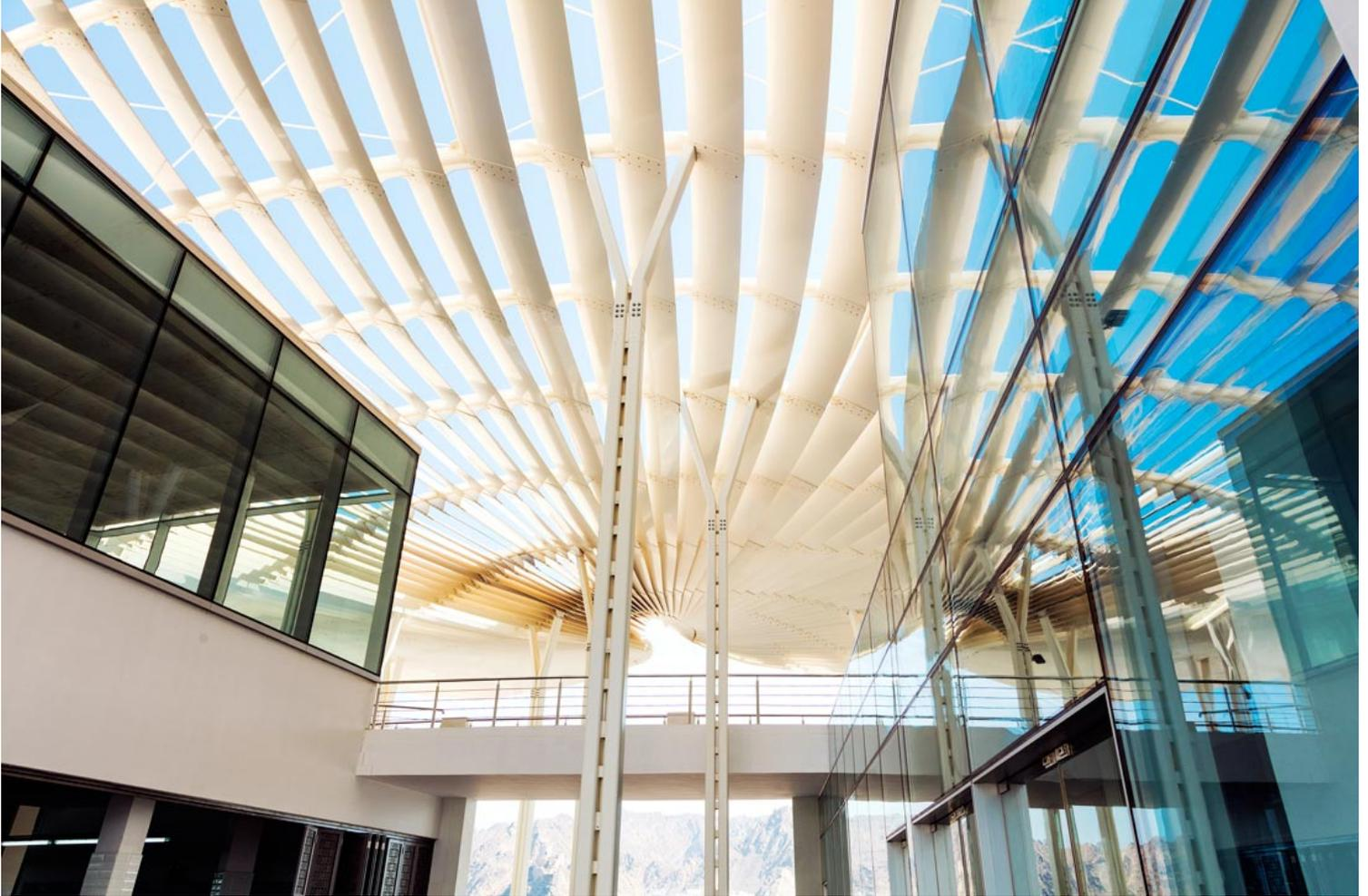
**At street level, the new market enhances the public setting by forming a dynamically shaded canopy, organizing the spaces beneath it. The canopy's form is derived from the sinuous flow of Arabic calligraphy. It follows the logic of a playful movement of light and shadow built from aluminum fins which provide shade, natural ventilation, and an ephemeral appearance. The complexity of the canopy roof contrasts with the simple solidity of the concrete structure below it.**
