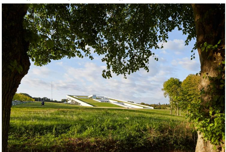
The green roof of the museum contributes to decreasing the energy consumption of the building. The roof reduces the overall need for cooling due to decreased heat absorption. Furthermore, the
