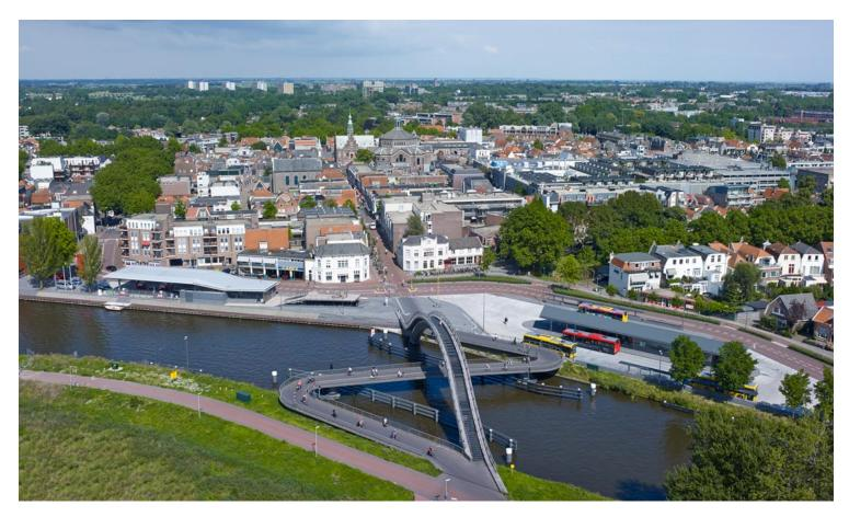
For this reason, the bridge separates bicycle and wheelchair traffic from pedestrian traffic. The bicycle bridge meanders over the water, which makes it long enough to limit the gradient.
