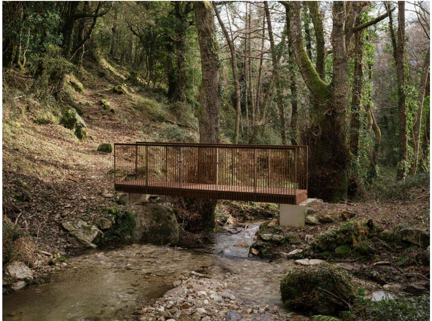
The purpose of the steel is to oxidize with time and weather so that the colors merge with nature and revoke an already-there object.
