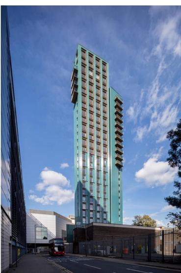
The building is arranged around a triangular stair and lift core. The building is composed of two wings, one facing east over the River Wandle and one facing south. All circulation spaces are naturally lit and ventilated and provide views in 3 directions. The residents lounge, entrance foyer,
