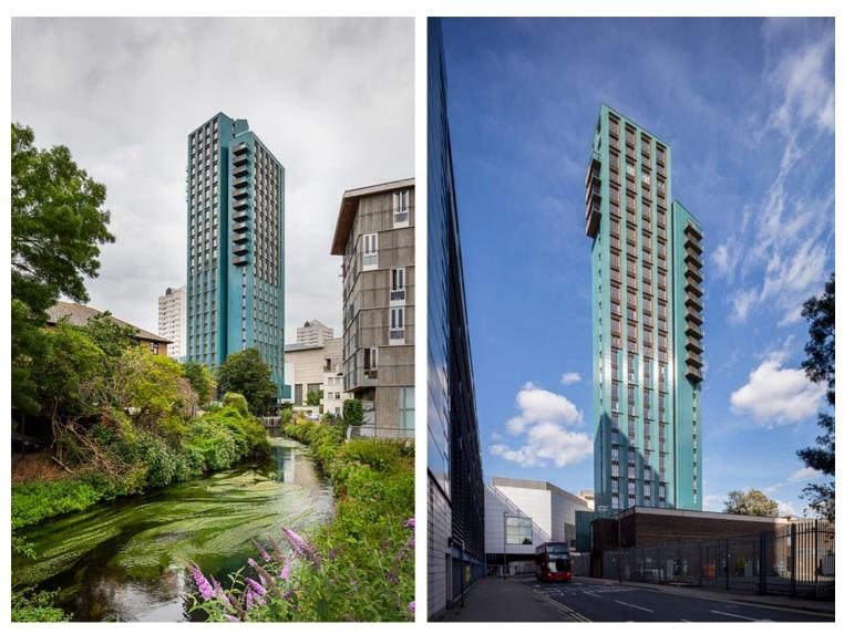
The building is arranged around a triangular stair and lift core. The building is composed of two wings, one facing east over the River Wandle and one facing south. All circulation spaces are naturally lit and ventilated and provide views in 3 directions. The residents lounge, entrance foyer,
