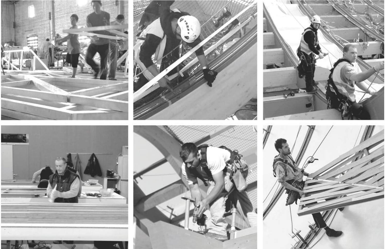
A collage of construction photos (clockwise from upper left): aluminum panel frames fabricated in China; installation of waterproofing extrusions; PVC installation; bamboo panels being installed; supporters being installed; and panel assembly.
