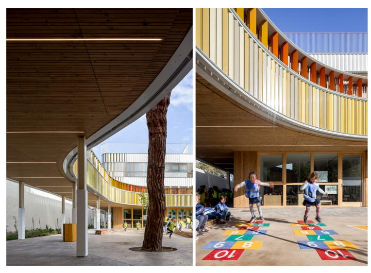
The image of the façade is derived from an envelope of vertical slats that run along the entire perimeter of the building. The position, orientation and separation of these slats has been studied to provide optimum solar protection, and they are highly efficient in their environmental and thermal terms and in durability. The play with colour and proportion is the result of a continuous dialogue with the client, who from the beginning wanted to include colour in the design.
