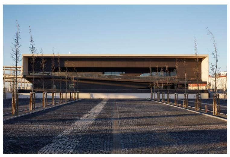
This sort of exoskeleton, which encircles the areas assigned to the terminal's program, is built of structural white concrete with cork – a solution specifically developed to reduce the building's weight, limited by the preexisting foundations. This solution stemmed from a concept by Carrilho da Graça originally developed for experimentadesign, the Lisbon design biennale, with a particular haptic quality, which lights up in the sunlight reflected on the estuary: the famous "light of Lisbon".
