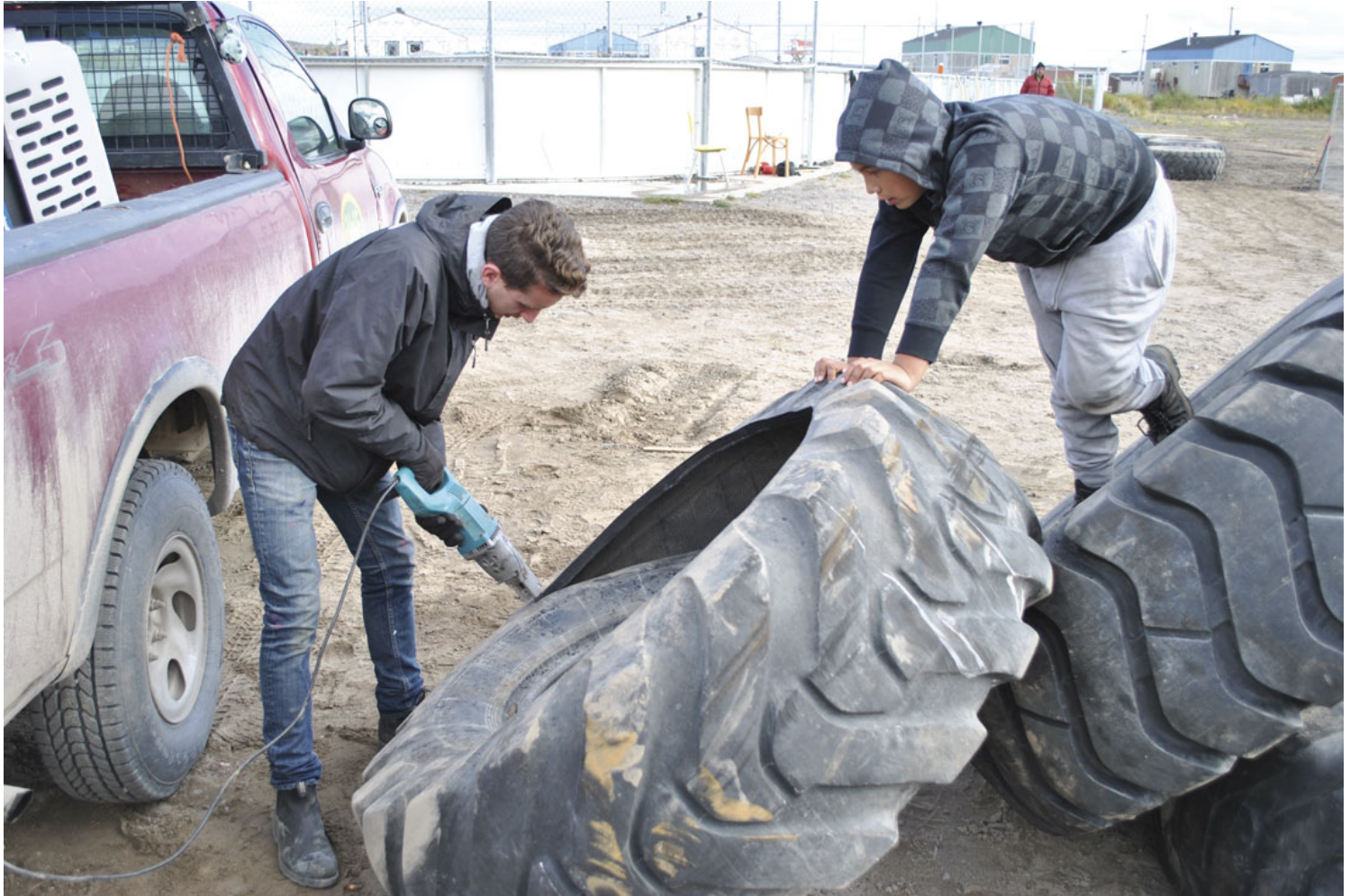
Modifying tractor tires for the base of the light beacon. Kuujuuaq, QC, 2017
