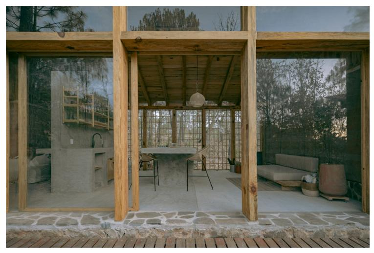
The structure of the design is based on monolithic, 40-cm thick loadbearing rammed earth walls. They sit on an elaborate stone foundation and support a ceiling of wooden beams, joists and tiles.
