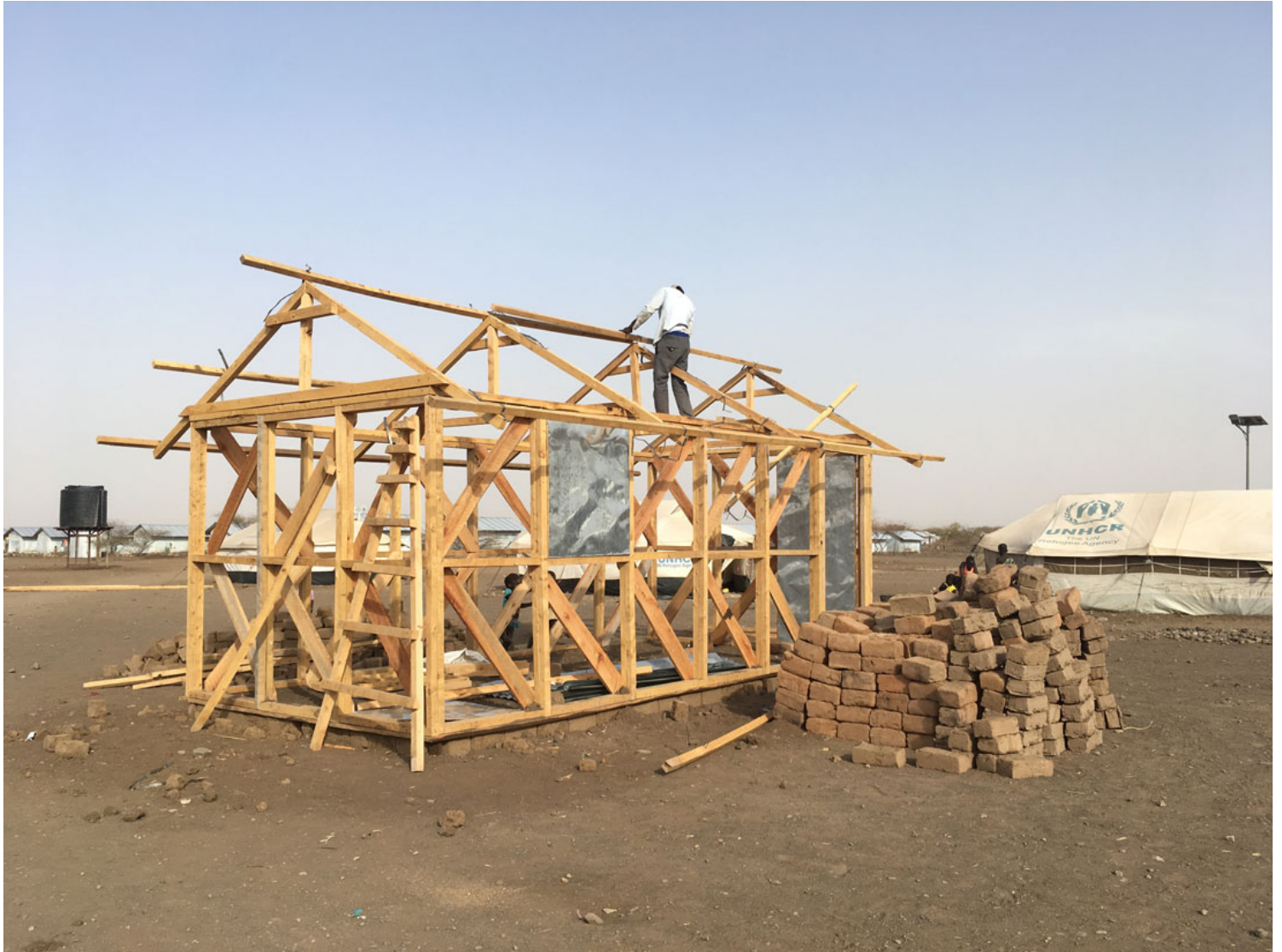
Completion of Timber Framework
