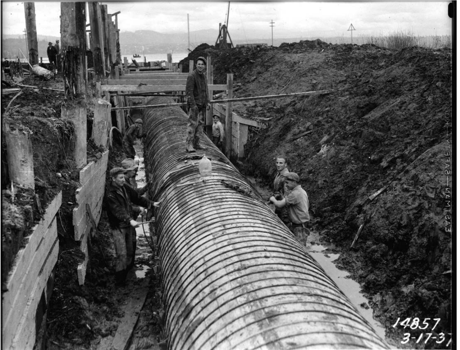
The quintessential image of job creation via infrastructure investment: WPA workers on the Henderson Street trunk sewer in Seattle, 1937. Photo via Seattle Municipal Archives.
