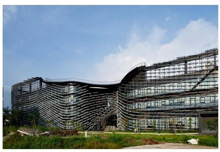
The fins are made of expanded aluminum sheet, creating a light-weight impression of the façade while allowing exterior views from the interior to some extent.
