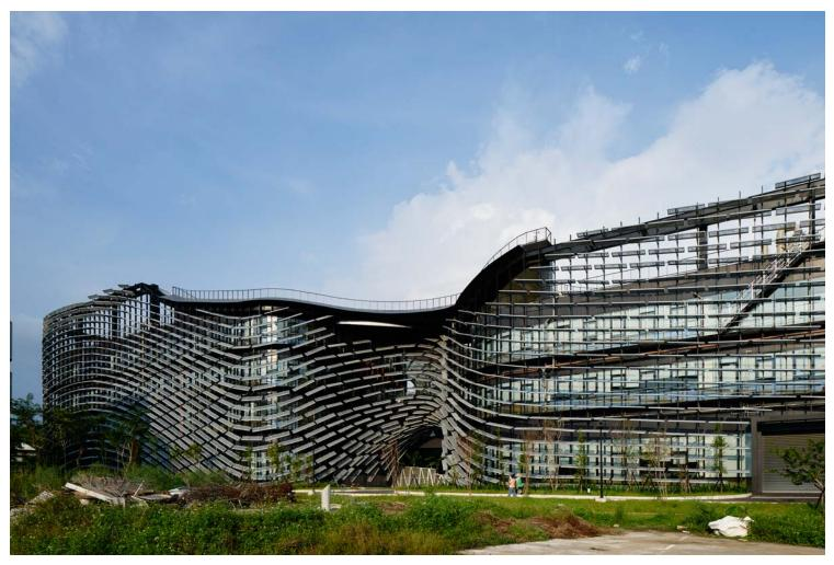
The fins resemble a school of fish- the fins are positioned at various angles, while as a whole creating a large flow and giving a dynamic impression to the building. The fins are made of expanded aluminum sheet, creating a light-weight impression of the façade while allowing exterior views from the interior to some extent.
