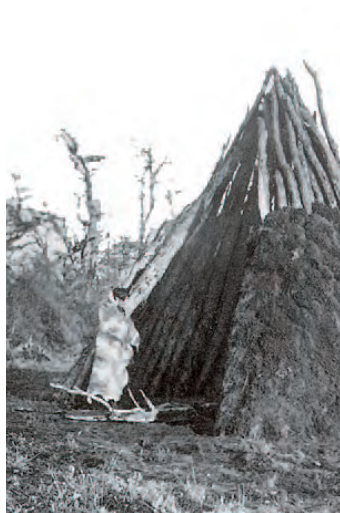
Hut built from linear elements forming cones. Ona culture.
