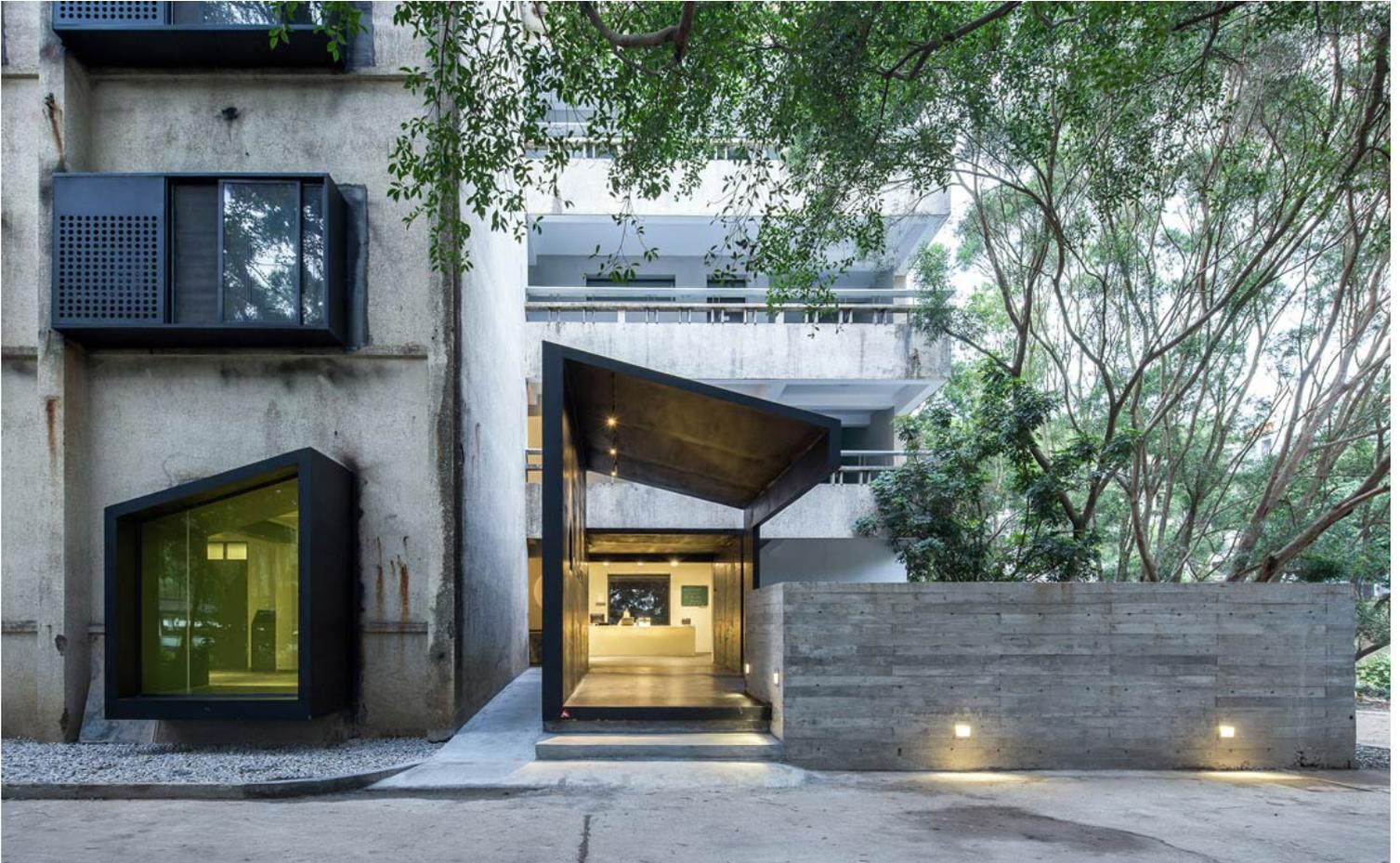
The renovation process consisted mainly of two spatial actions: first, equipping the central corridor with new hotel infrastructures to serve the new living units; and, second, installing a sequence of prefab steel boxes to generate openings in the existing façade, creating a more dynamic interaction between the building and the surrounding nature.
