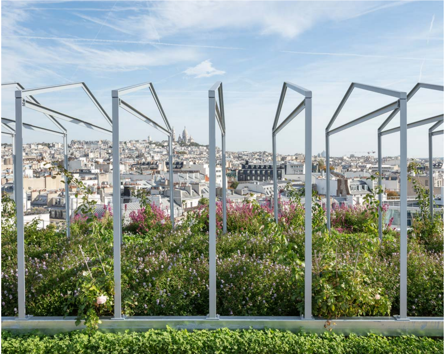
Rooftop Garden, Grand Central Saint-Lazare, Paris, France, 2019. Photo by Luc Boegly.
