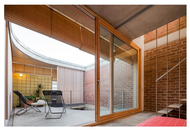
As for the materials, exposed concrete and uncoated brick were chosen, together with unpainted wooden joinery, continuous mortar floors and exterior cork cladding. To avoid altering the rough appearance of the materials, surface treatments such as waxes, oils or colorless Lasur were used.
