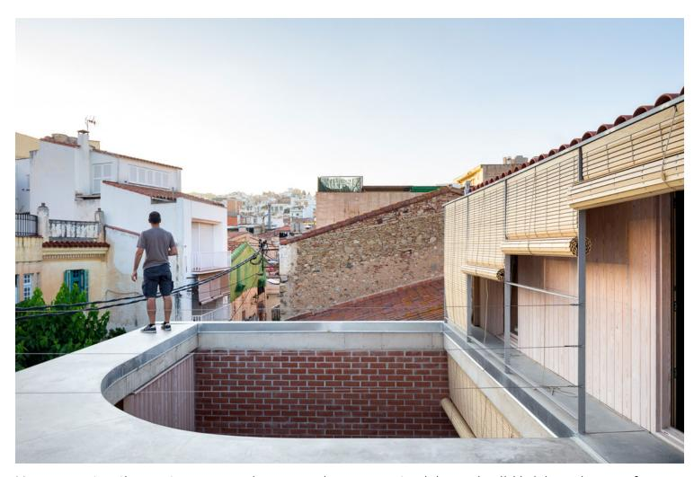
Heavy construction systems were chosen, such as concrete slabs and solid brick enclosures for their thermal insulation properties, all playing a key role in the building's desired passive performance. This inertia cushions and lags the daily and seasonal thermal oscillation and is especially suitable in a permanently occupied building: in this case, a home that also incorporates a workspace.
