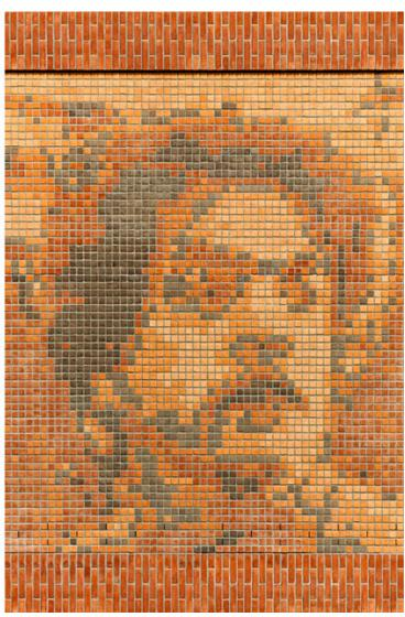
The images are elaborations on the base of archive photographs. Details within the photographs have been cropped in order to match the façade panels' proportions. These portions of photographs have been then reduced to a number of pixels equal to the number of bricks contained in the panel and then processed and subdivided in six colors, so that to each brick in the façade panel would correspond to a pixel of the elaborated image. The result of this process was a matrix with numbers
