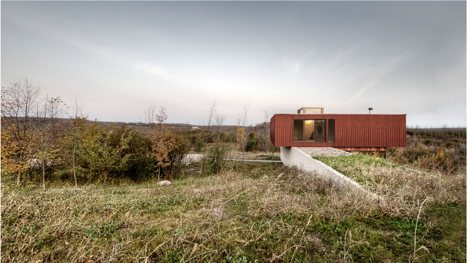
View of the second floor family room walkout to the landscape.
