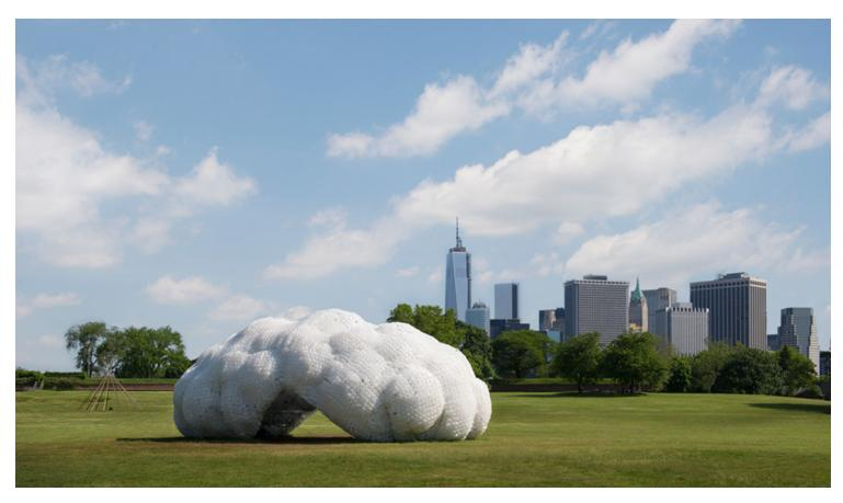
A series of "pillows" made from one-gallon jugs form the exterior, while 16- and 24-ounce water bottles line the interior. A curved aluminum diagrid frame provides structural integrity and creates a small seating and dreaming area for 50 people at the base. The water bottles were filled with varying amounts of water and organic blue food coloring to provide ballast so that no foundation was needed.
