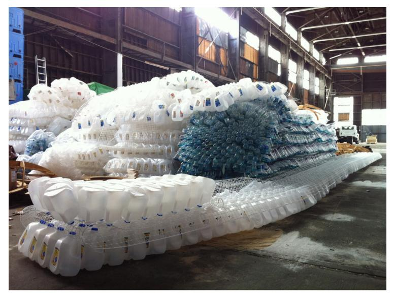
All of the building components can be easily broken down and transported, including a lightweight aluminum diagrid: a simple way to provide structural integrity without relying on heavy steel beams or larger support systems. Rather than employing high-tech fabrication techniques to turn the bottles and aluminum into cladding and structure, the design team created a simple, repetitive, cost-effective system of connections, in order to quickly and easily assemble this free, public structure.
