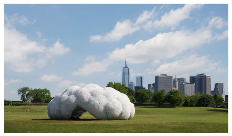
A series of "pillows" made from one-gallon jugs form the exterior, while 16- and 24-ounce water bottles line the interior. A curved aluminum diagrid frame provides structural integrity and creates a small seating and dreaming area for 50 people at the base. The water bottles were filled with varying amounts of water and organic blue food coloring to provide ballast so that no foundation was needed.
