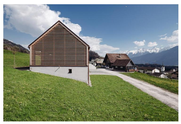
The ground floor is cut into the slope and constructed in a solid construction with building component activation. In this way, the solar energy is stored in the building mass. A wooden building with a saddle roof in copper roofing stands on top of it. The floor plans play with density and generosity. The upper floor has a western terrace and an open gable with gallery.
