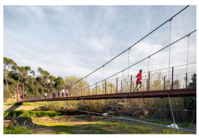
The footbridge owes its structural integrity to two sturdy pillars, towering at a height of 9 meters on each end. These pillars anchor the bridge, while two primary steel cables, known as catenaries, ensure its stability and durability. The footbridge incorporates additional crosswise cables beneath the deck, enhancing its resilience against extreme weather conditions such as strong winds and storms, while minimizing vibrations.
