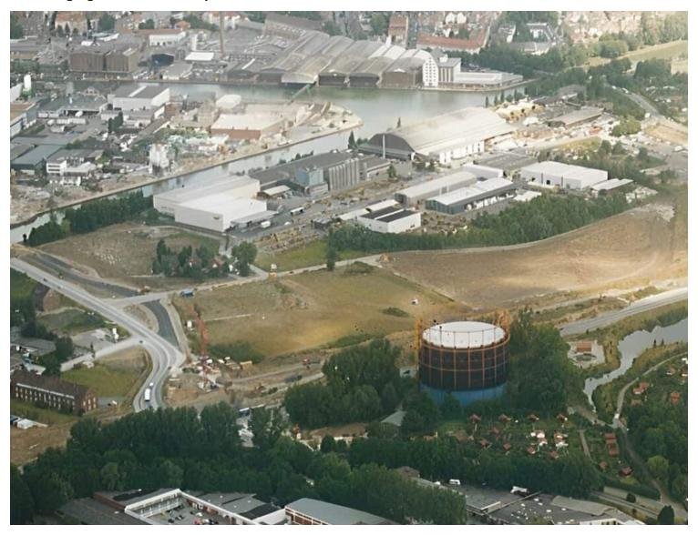
The Gasometer is composed of a closed steel plinth about 12 meters high, topped by an open steel structure surrounding a telescopic cylinder to store natural gas. The steel frame and plinth are
