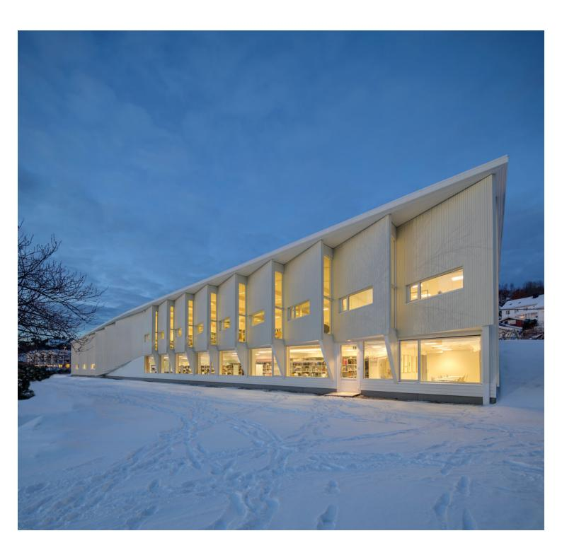
An existing building on the site, together with the budget, formed a limited framework for the project. However, this limitation was looked upon as a positive; the old structure is partially kept and acts as foundations for the new light timber structure. The compact volume of the building has a rational timber structure. The timber frames are placed with a spacing of 3 m on top of the existing concrete building.
