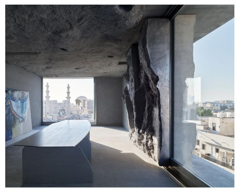
On the interior the sand casting is repeated in the concrete floor slabs, which are made in the same way. Large shutters can be moved in front of the windows. The shutters (and the entrance door) are made out of sand casted aluminum with the relief facing towards the interior. Contrary to the concrete elements, the aluminum sand casts are hollow. The interior of the casts can be seen through the windows.
