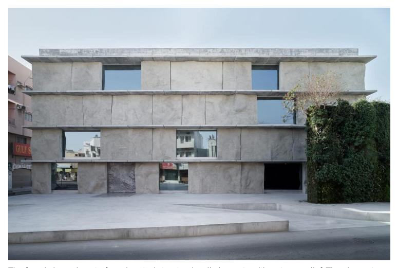
The façade is made out of sand casted structural wall elements with a strong relief. The elements are cast on the ground next to the building. Each cast results in a unique imprint on the element. At the windows and the corners of the building, the relief is visible, like a geological cut in the ground.
