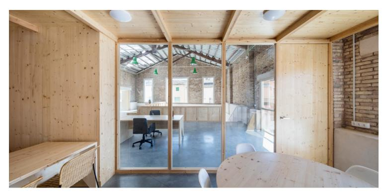
In the first place, the main structure of the new workshop has been designed following the main axes of the existing building structure. The preservation of the orientation and module of the structure of the old building orders and links the two buildings and at the same time allows the oblique side of the trapezium to be resolved in the same way, absorbing the geometric deformation in the structural section of the main façade.
