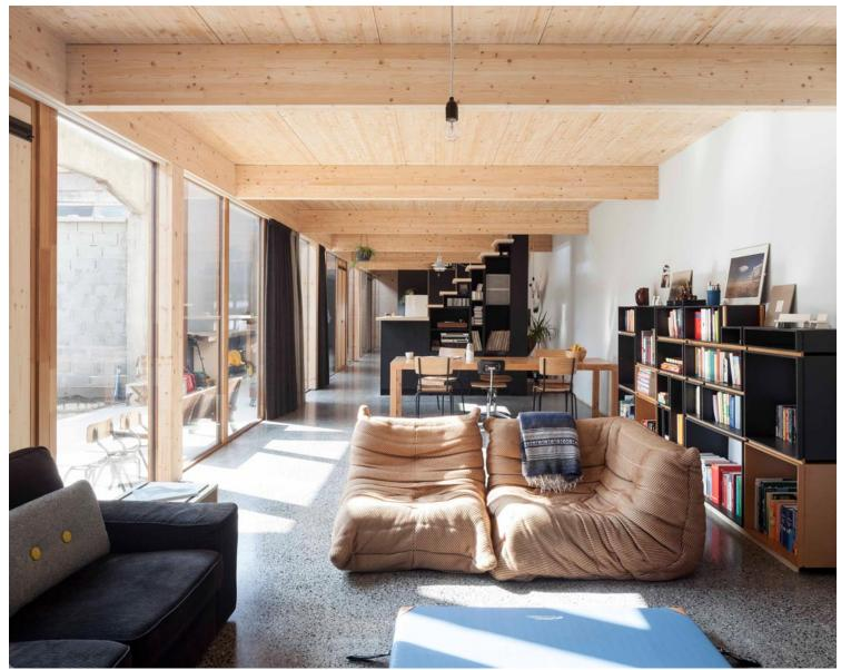
The design leaves the existing structures intact and adds a third, light wooden structure. A compact, two-story residential volume is placed under the roof of the high shed, pushed to the side walls. The slabs of the concrete structure are removed to create a walled garden. The existing concrete structure is preserved in the garden and is copied in the wooden structure of the house.
