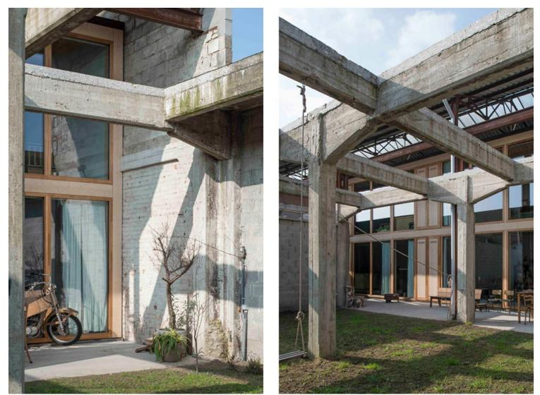
The site has been refurbished with a cluster of new residential units and small workshops around a central square. The client owns a portion of the site, which consists of a concrete structure adjacent to a double-height steel structure.
