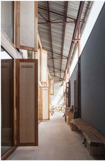
The design leaves the existing structures intact and adds a third, light wooden structure. A compact, two-story residential volume is placed under the roof of the high shed, pushed to the side walls. The slabs of the concrete structure are removed to create a walled garden. The existing concrete structure is preserved in the garden and is copied in the wooden structure of the house.
