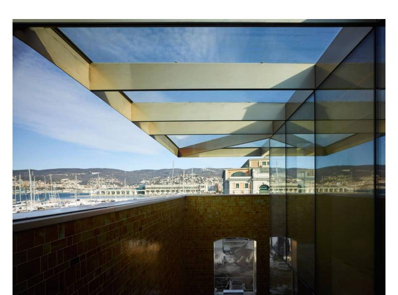
Their redevelopment and conversion plan protects the existing building while maintaining absolute respect for its city setting. The plan leaves the original volume unchanged, placing within it a new, all glass architectural structure connected to the existing perimeter by walkways suspended over the water.
