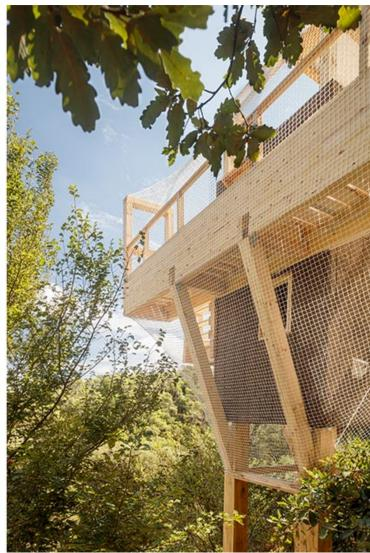
The surrounding net, which takes influence from a hunter's nest, was designed digitally and then woven by hand. The net is intended to better camouflage the construction by allowing plants to grow across it, thus further merging the structure with the forest in order to hide it from the surrounding wildlife.
