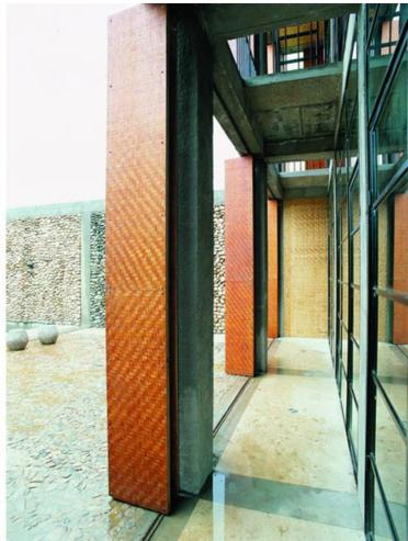
Therefore, use of the alien (concrete) remains a minimal and distinct element whereas use of the local (stone and wood) is maximized. The stone is treated differently depending on where it occurs within the didactic realm of the concrete frame. This collision of rough, organic materials with highly regulated and spare form gives the house an ephemeral quality encased in distinctly modern
