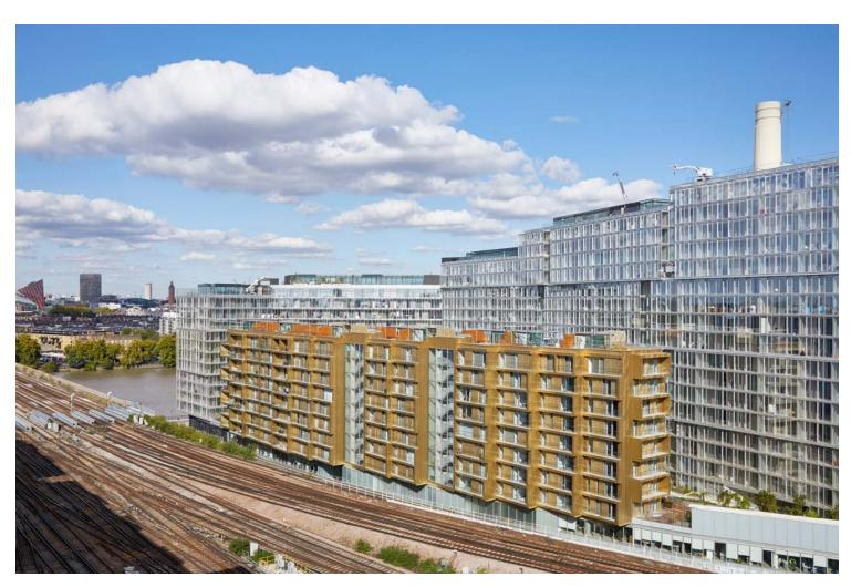
Faraday House is formed from a series of stacked apartments that shift in response to the curve of the tracks, generating an interesting form of projecting and recessed boxes. The 8 storey building is clad in copper alloy; a bright, folded metal that reflects a hand-worked aesthetic and gives the building a striking identity.
