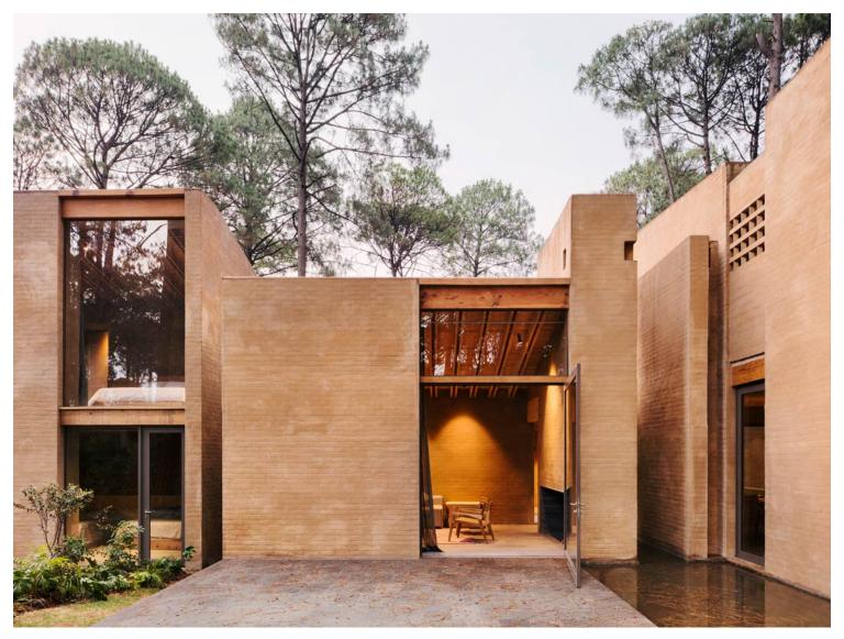
The materials are from the region: brick, wood and soil. By reusing the soil culled from the site to cover the walls, the five buildings have a warm, natural and terracotta colour finished.
