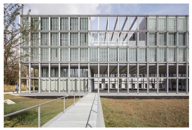
Inscribed in a 80 m x 80 m square, the building is an open, welcoming and urban place, but it borrows the notion of an interior landscape from the shape of the cloister. The continuous 3.05 m x 2.10 m grid made with HEB profiles measuring 24 cm x 24cm, weaves the entire project and draws its architecture.
