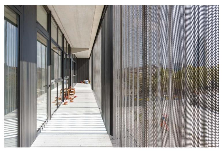
On the façade, the use of large steel panels provided the building with a clear-cut urban scale, while simplifying the assembly and later maintenance. This latter aspect was present in all of the design decisions; in this respect, we chose materials with a long useful life or elements that could be easily repaired.
