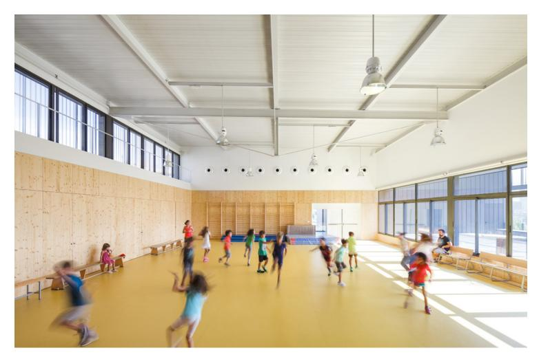
Given the subsoil's characteristics, the building's weight was reduced as much as possible to avoid the need for a deep foundation. The building consists of a double block connected by a central space with porticoes every 7.5 metres to adapt to the dimensions of the classrooms. The classroom spaces are covered by one-way slabs based on lightweight concrete shuttering slabs, while a solid slab that ties the whole complex together covers the remaining spaces.
