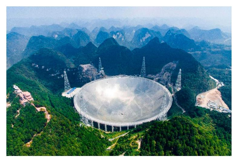
FAST: Five-hundred-meter Aperture Spherical radio Telescope - the world's largest filled-aperture radio telescope. Photo taken on July 3, 2016, the day the huge dish's last panel was installed. Image: © Xinhua
