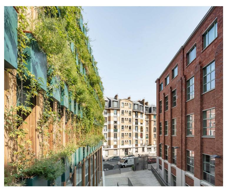
Thus, 290 large planters punctuate the windows of the façade, with an average of 14 planters per unit, which, along with the shared allotment, equates to 10 m2 of soil per apartment!
