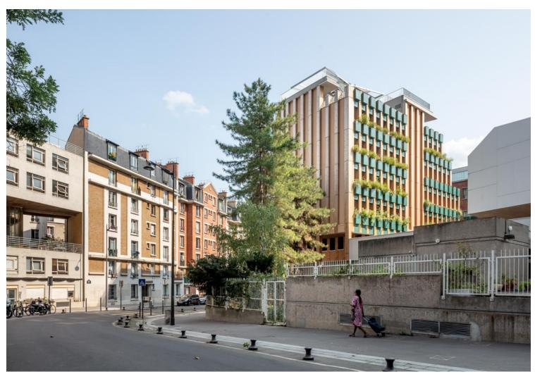
With regards to materials, the project established the principle of 'the right material in the right place'. The result is an optimized combination of concrete, timber and metal.
