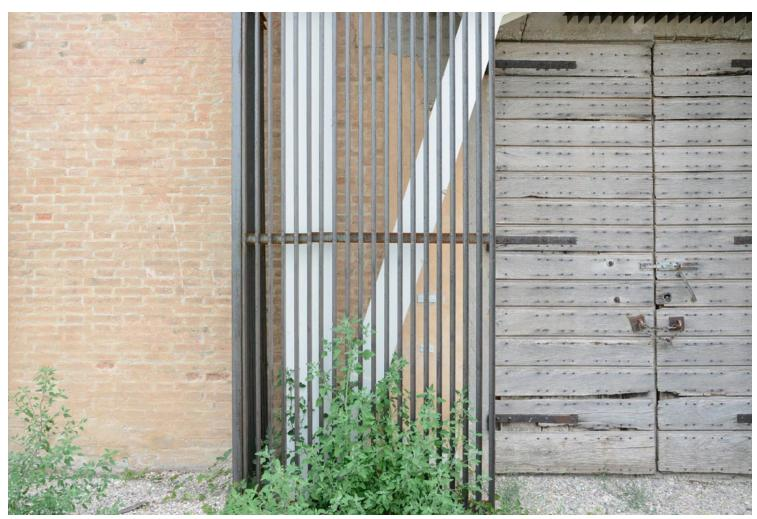
The new covering in corten steel links the restored façade with the new volume, while revealing the stratification of the interventions. The perception of the façades is dynamic and changes from the different angles, emphasizing the historical façade, the relationship with the contemporary intervention, or the strength of the oxidized steel.
