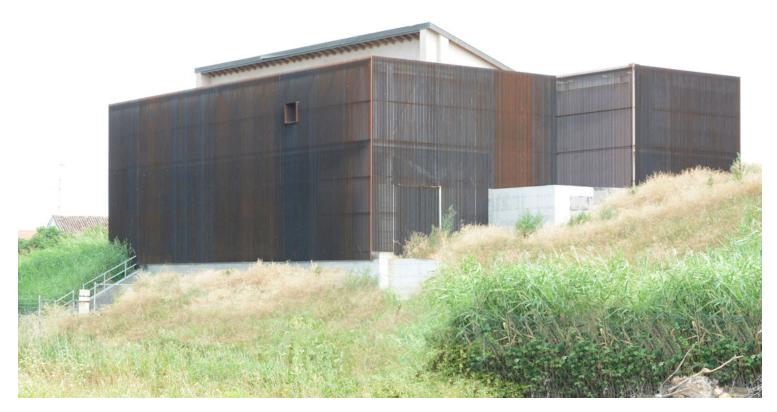
A new reticular steel structure with polycarbonate wall replaces the volume that was destroyed; inside there is a polyvalent space which houses the environmental learning center for the Secchia River Park. The construction materials for the new volume are concrete and steel in order to stand up to the pressure of water and guarantee reversibility.
