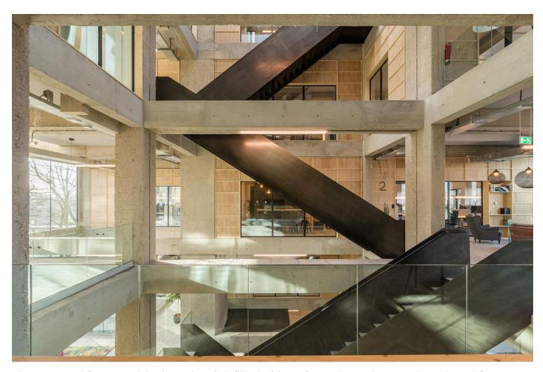
The structural framework in the atrium is infilled with perforated wooden panels and steel frames. In addition to their acoustic function, the walls also incorporate various functions such as the kitchenettes, library, storage and displays.
