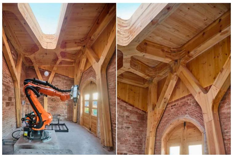
The students of the 2023/24 class of MAEBB worked with an integrated system that spanned from scanning the trees felled on-site, to orienting and programming the robotic cuts, and assembling the structure in the forest. The result is a space that embodies a choreography between human gesture and digital code, matter and intent.
