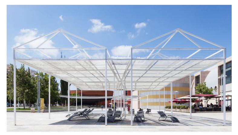
"Cloud Seeding" creates boundaries between sun and shade that are dynamic, responsive, and fragmented. These boundaries are the result of thousands of lightweight balls, or "seeds," in motion on a fabric mesh ceiling. The "seeds" are made of PET plastic and are recycled content from plastic water bottles.
