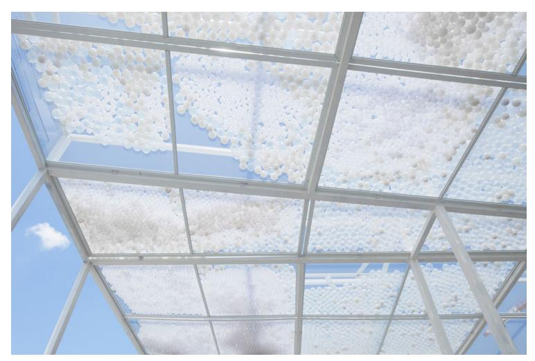
"Cloud Seeding" also transforms a building type ubiquitous in Israel's agricultural landscape: the greenhouse. In this context, the greenhouse consists simply of a structural frame (without wall and roof panels) that supports the mesh ceiling and balls. The agricultural greenhouse has been re-appropriated as a plaza pavilion for culture, leisure and public events – all informed by the changing patterns of the weather overhead.
