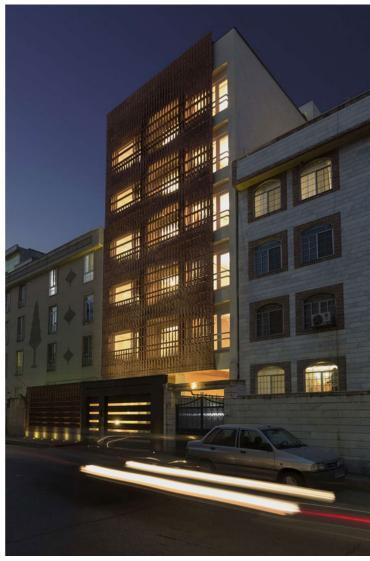
Rotating the bricks provided the opportunity to have various degrees of openings, and the rotation angles are precisely adjusted through a dialogue between inside and outside taking into account sun direction, daylight and the level of distraction from adjacent apartments. Despite the complex form of the façade, the construction process was easily executable by workers through simple instructions prepared by using a coding system.
