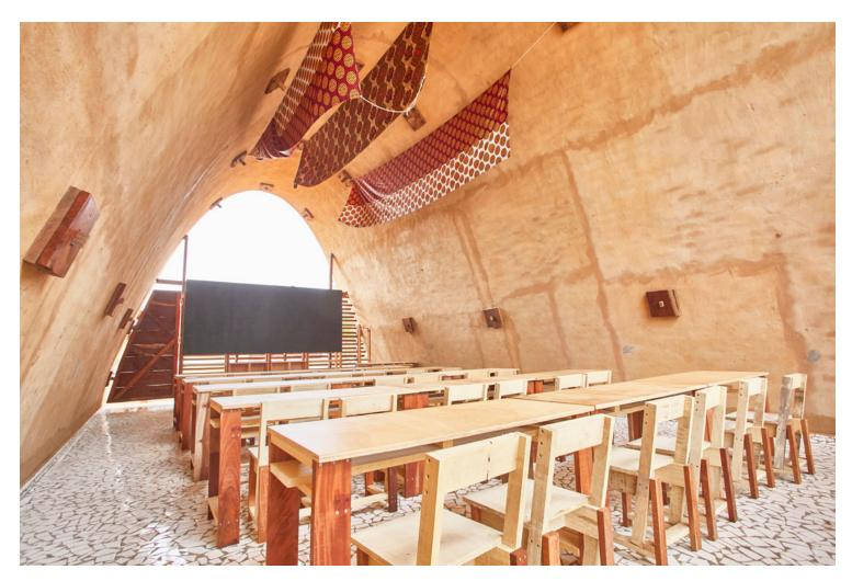
The space that covers each of the Awlas is enclosed by two wooden lattices that allow lighting and air circulation from north to south. Thanks to this ventilation and the porosity of the clay, the cooling evaporator effect is achieved so that there is no need to resort to mechanical air-conditioning systems. The vaults are covered by a corrugated iron sheet to prevent direct rain from falling on the clay and to provide a shaded air chamber.
