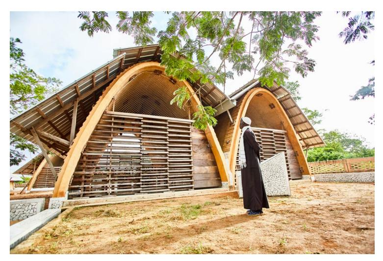
The school is understood as a system that can be adapted over time; it is comprised of modules that can be arranged within a grid, thus allowing the school to grow by building new modules, called Awlas, as required.
