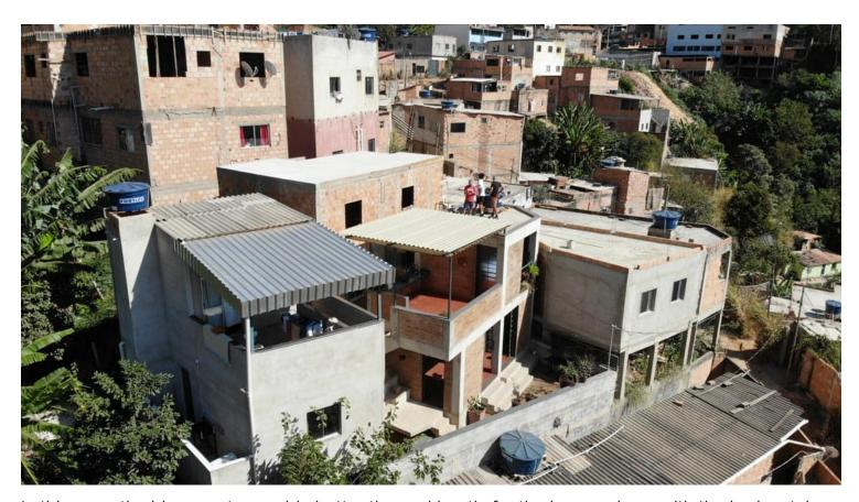
In this case, the idea was to provide better thermal inertia for the house, since, with the horizontal layout, the thickness of the wall corresponds to the longer edge of the brick. In addition, we explored different ways of using the brick as a modular element: in some cases, it forms a lattice, and in others it is combined with concrete blocks for structural purposes.
